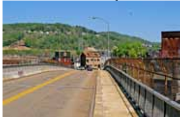
Lower Herron Avenue Bridge
