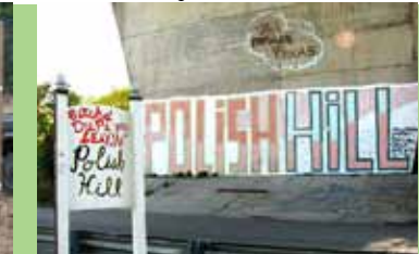
Bloomfield Bridge Portal
