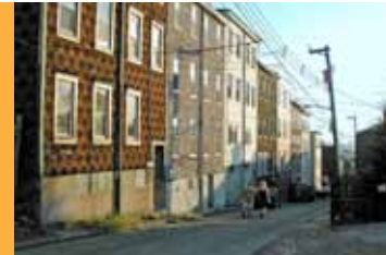
Pulawski St. Rehab
