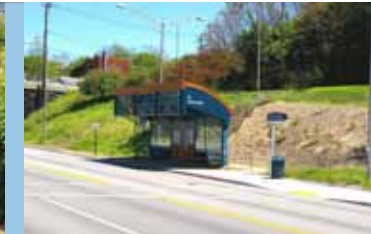
BRT Station at Lower Herron
