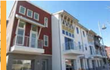
Live Work Garage Exterior
