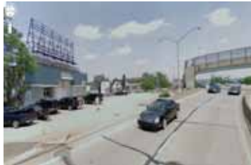
Pedestrian Bridge- Bigelow Boulevard
