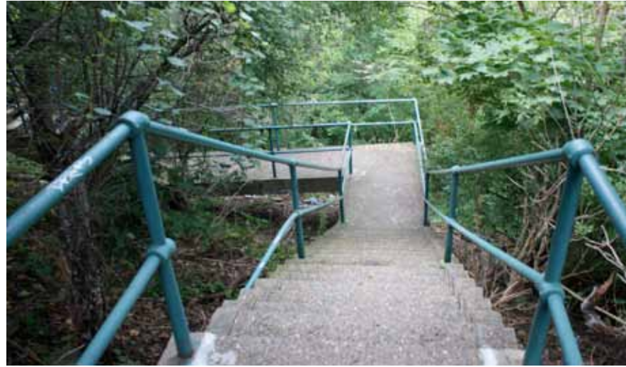
Public Stair Improvements
