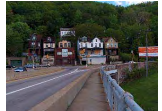
62nd St Bridge Gateway: neighborhood entry
