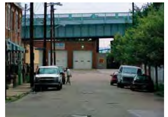
Willow Street Under 40th St. Bridge
