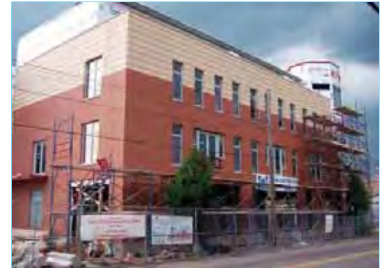
New loft construction: 35th and Butler St.
