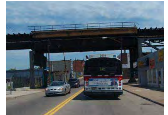
33rd St. Train bridge entry to the neighborhood
